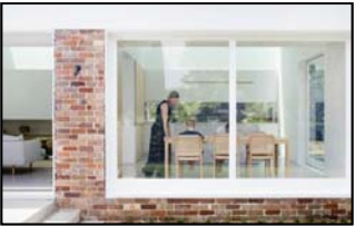
OFF-WHITE METALLIC POWDERCOATED ALUMINIUM & CLEAR LOW-E GLAZING
